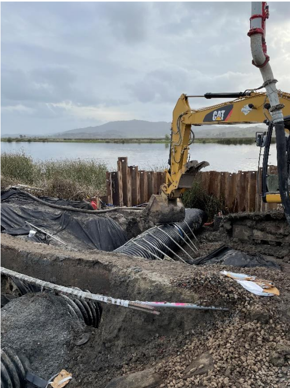
Figure 6 – New 48-inch outlet pipe installation
