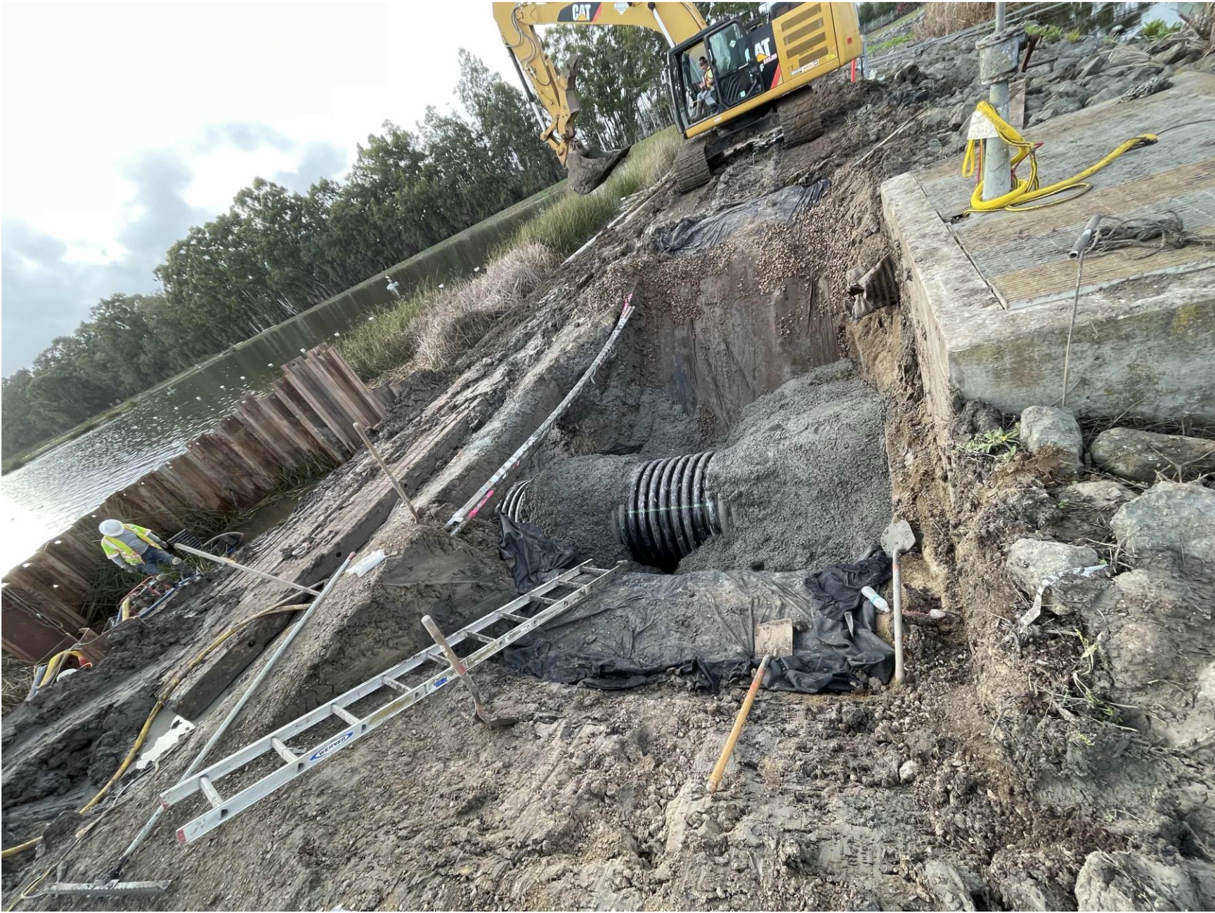
Figure 5 – New 48-inch outlet pipe installation
