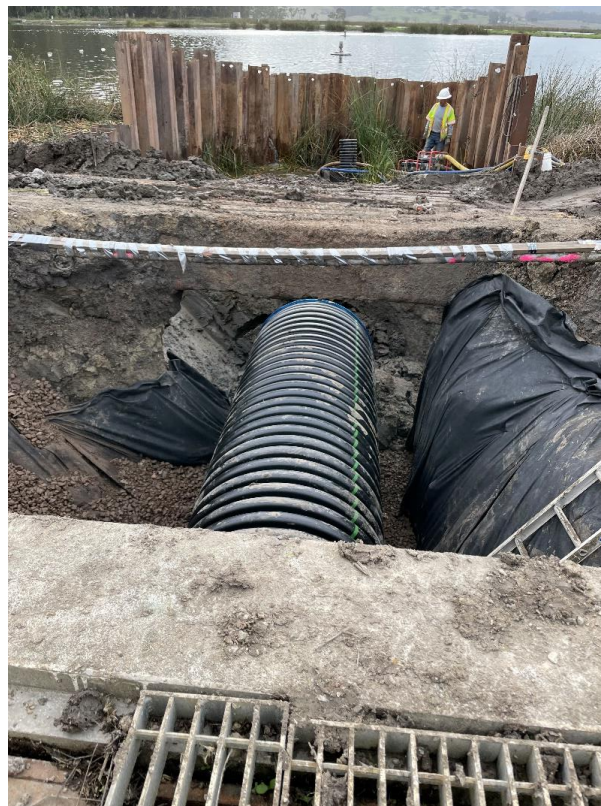
Figure 4 – New 48-inch outlet pipe installation
